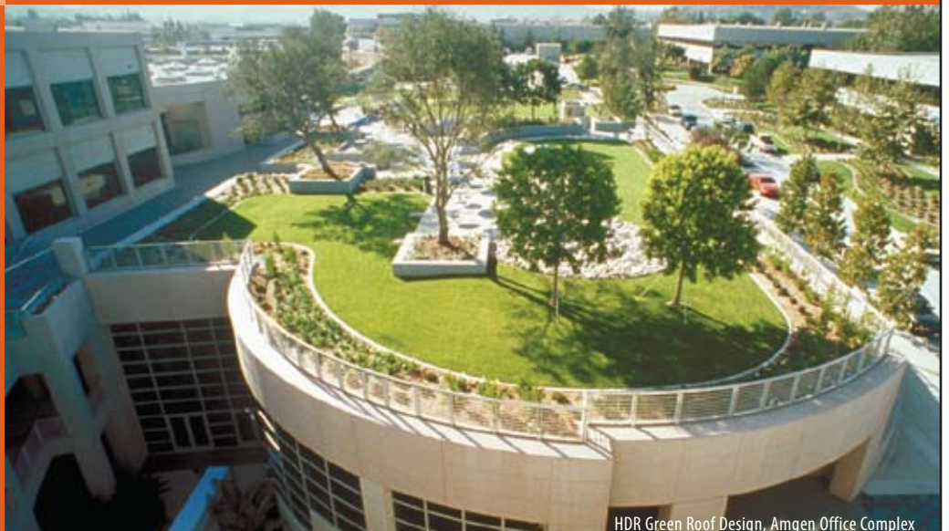
HDR Green Roof Design, Amgen Office Complex
