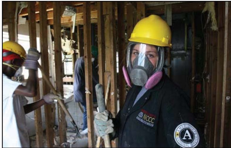
An AmeriCorps member inside a house damaged by Hurricane Katrina in Louisiana.
